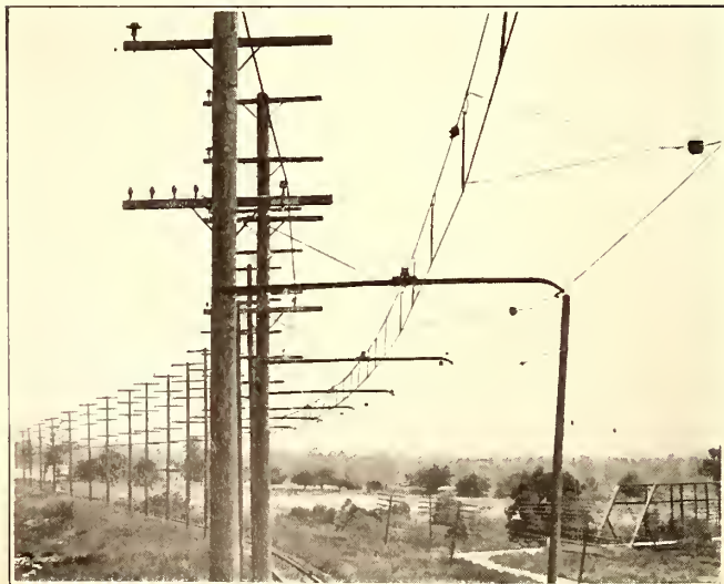
VIEWS ON SAN BERNARDINO LINE OF PACIFIC ELECTRIC RAILWAY SHOWING OVERHEAD CONSTRUCTION WITH STEEL CONTACT WIRE
